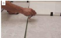
It is not necessary for general installations, but in areas with large and continuous water spills, it is recommended to apply our Clic Seal sealer. This should be applied to the tongue side of the click system.
