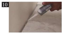
Once the profiles have been measured and cut, it is time to apply flexible silicone around the perimeter between the floor and the wall, as well as between the planks which forms the expansion joint. After completing this step, the aluminium profiles can be installed.
