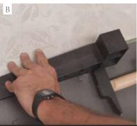
The installation can be done without the help of any tools, although if desired, special mounting wedges can be used (we recommend the FAUS ACCUTITE INSTALTION KIT).
