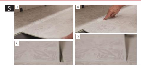
Start installing the second row according to the design pattern chosen. For example, for the design shown on the images, it should be cut to match the bevels indicated on each tile (approximately 50% of the plank from the previous row). In the case of a wood or stone design which allows it due to their structure, you can use the last piece from the previous row if it is longer than 40 cm.
